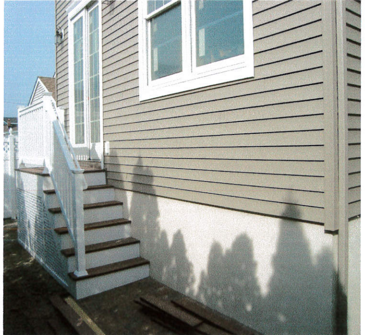
Rear View Date Taken: 11/10/2009
