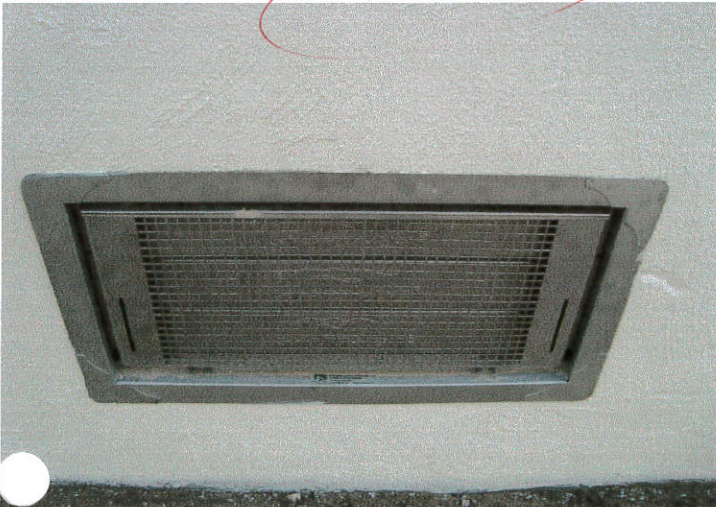
Vents (5) Date Taken: 11/10/2009- All 5 vents are Smart Vents Certified for 200 S.F. Each or 1,000 S.F. Total
